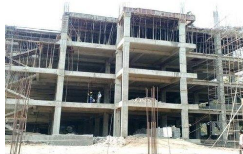
Plate 1. Typical RC frame building [7]
